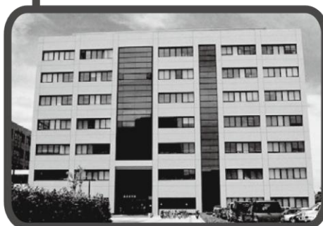
General Research Building
